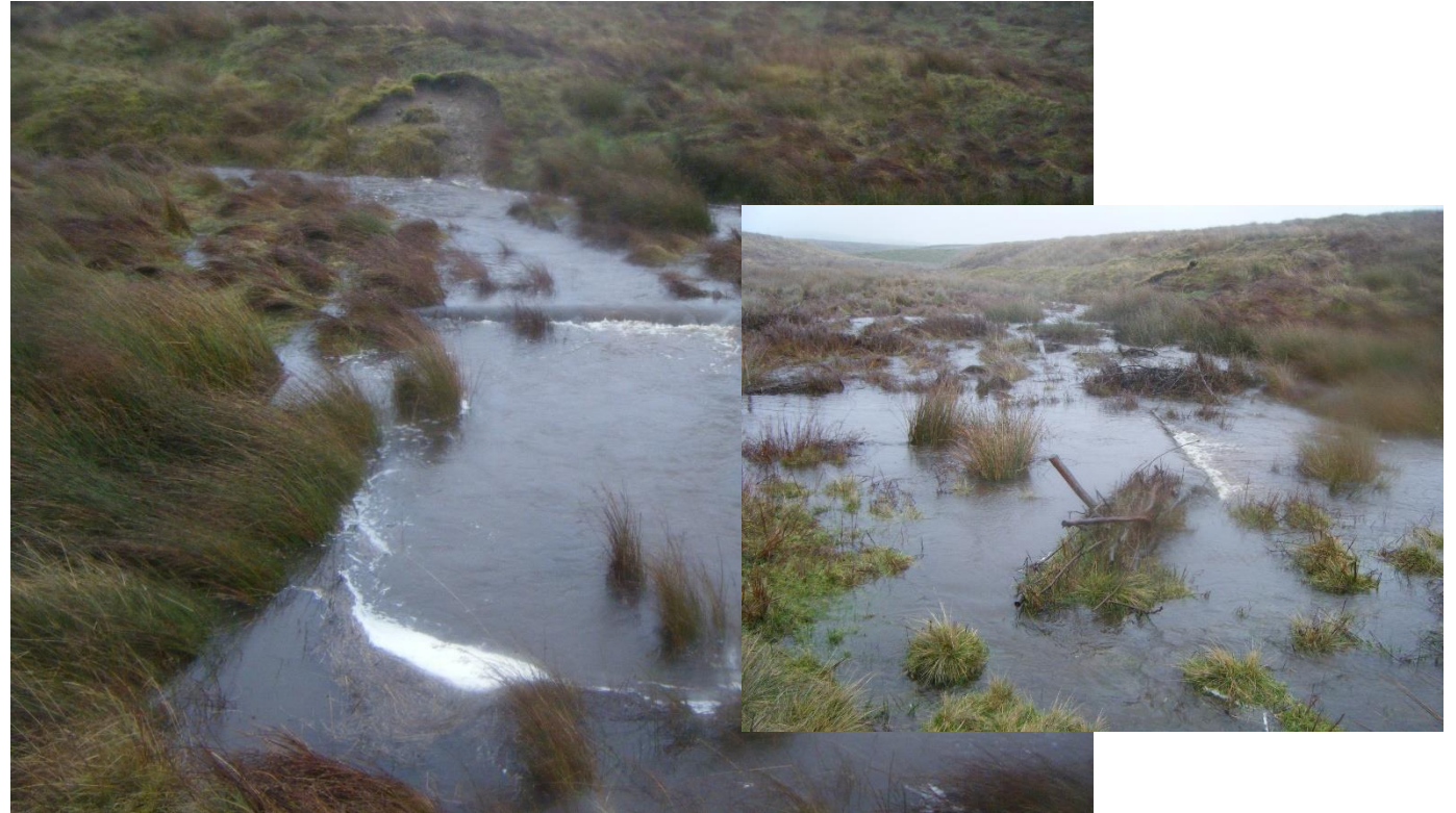
22-12-2014 Pont Gallon Burn Leaky Dams
